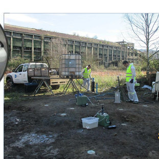
Figure 2. Spanish pilot test works execution
