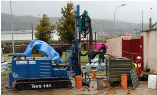
Injection at Spolchemie pilot site 1 (VEGAS/USTUTT)
