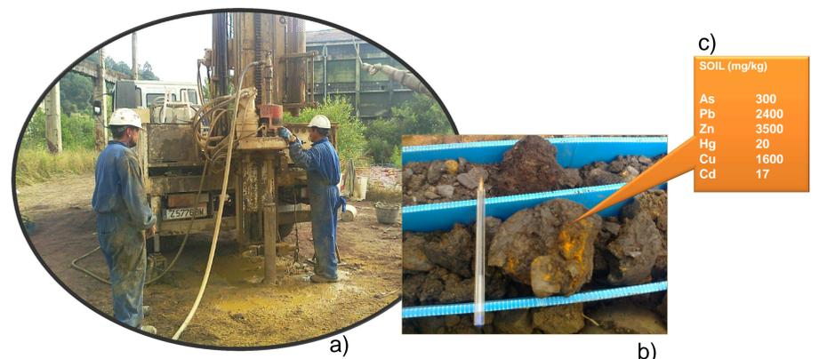
Figure 4.a) Diamond core drilling works, 4.b) pyrite ashes in madeground and 4.c) heavy metal content
