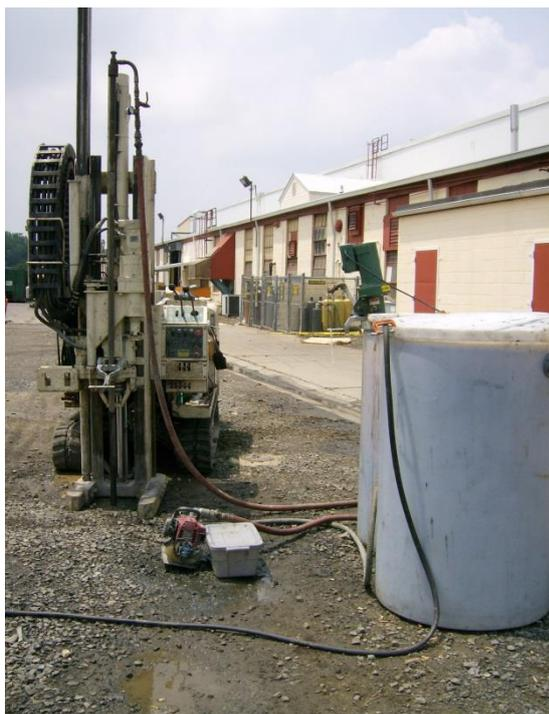
**Figure 2:** Direct Injection of nZVI in the Field at the Trenton Facility, New Jersey (Photo courtesy of Geosyntec Consultants)
