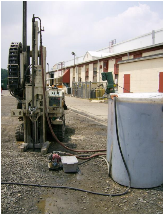
Figure 2: Direct Injection of nZVI in the Field at the Trenton Facility, New Jersey (Photo courtesy of Geosyntec Consultants)
